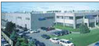
Montreal, Canada Velan Inc., Plant 2 and 7
