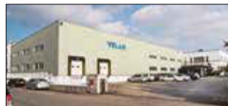
Ansan City, South Korea Velan Ltd., Plant 2
