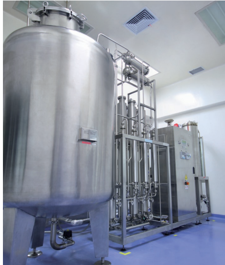
Flow measurement of demineralized water
