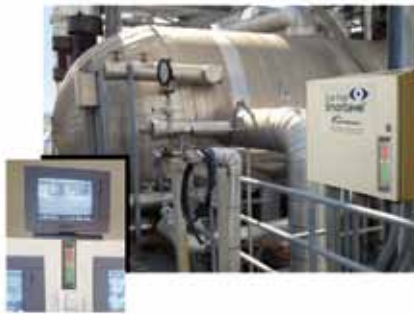
Eye-Hye® SmartLevel™ Local and Remote Indicators
