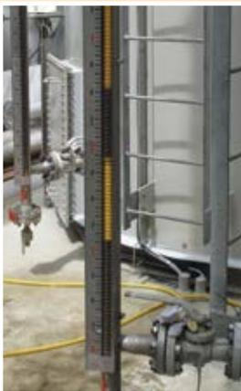
Weak magnetic coupling between the flags and float magnetic field can lead to missed flags and unreliable indication. Operator must manually “reset” the flags or wait for the level to cycle.
