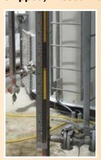
Weak magnetic coupling between the flags and float magnetic field can lead to missed flags and unreliable indication. Operator must manually "reset" the flags or wait for the level to cycle.
